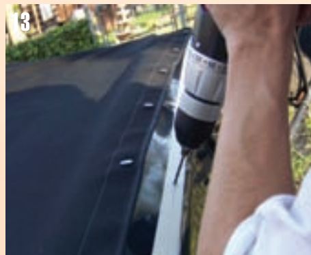
13 The measurements better be correct as it is time to drill holes. Using a 1/8" drill bit I carefully drilled the holes. Then I removed the masking tape.
