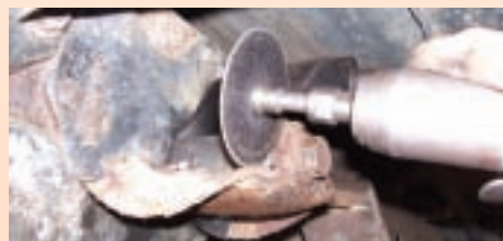
Full Force had been the victim of a flood at one point resulting in major rust under the truck. Here, a rusty bolt holding on the rear leaf spring bracket is cut off. It is replaced with a bolt from the Ford dealership. While the hardware to replace all the rusty bolts removed during this setup could have been found at an auto parts store or a fastener shop, the dealer was able to provide precisely the right high quality hardware taking the guess work and hassle out of hunting down the right size bolts.
