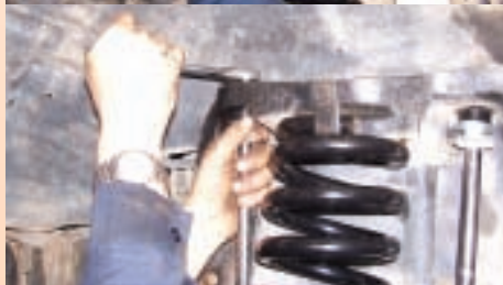
The new, taller shock absorbers are installed.
