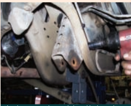
After disconnecting the pivot bolts and bushings, the entire TTB axle housing is lowered and the stock, TTB pivot brackets can be removed.
