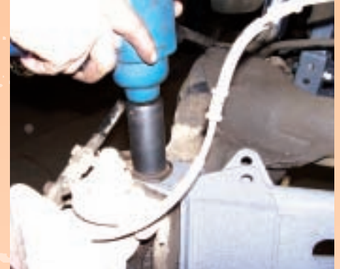
The new extended radius arms are bolted onto the axle.
